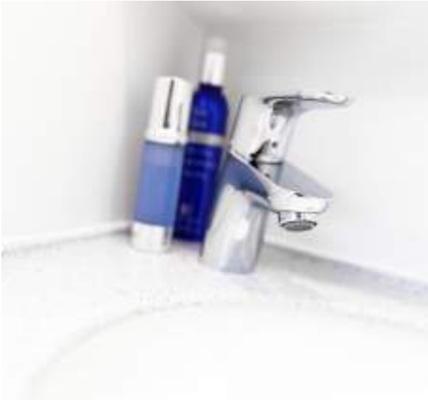
The worktop overlaps the sink, in order to prevent water from splashing up in a seaway
