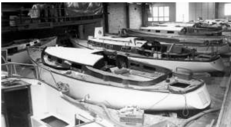
In the early 70s: A mix of GRP and wooden superstructures
